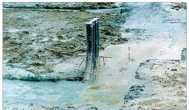
Energiebocht in fundering in volle grond
